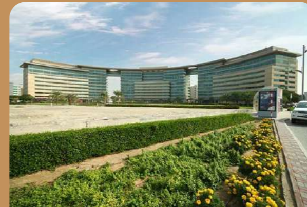
Al Hudaibah Awards building- Dubai
